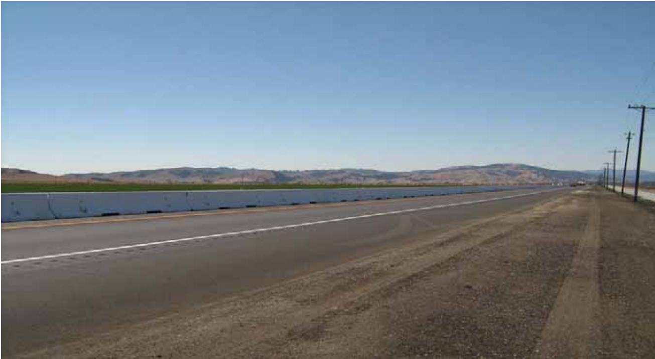
Hwy 25 Northbound with K Rail and Final Stripe (Finished Product)
