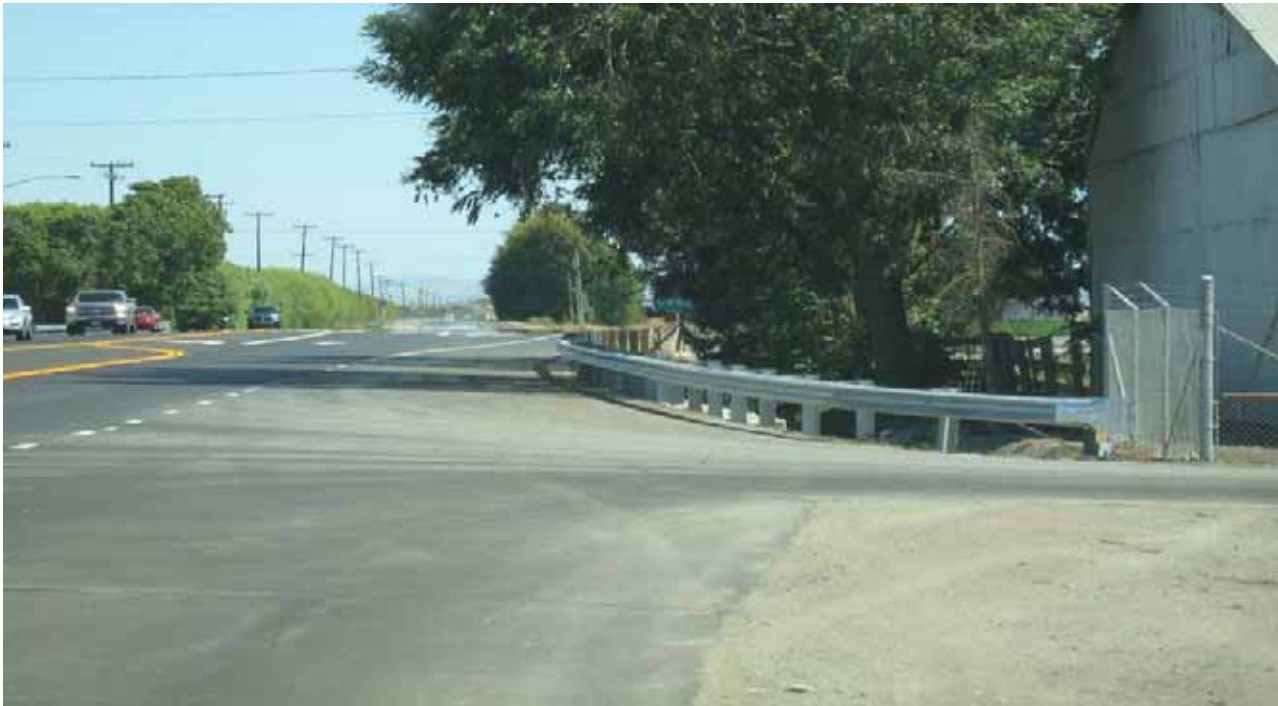
Hudner Ln with new Metal Beam Guardrail
