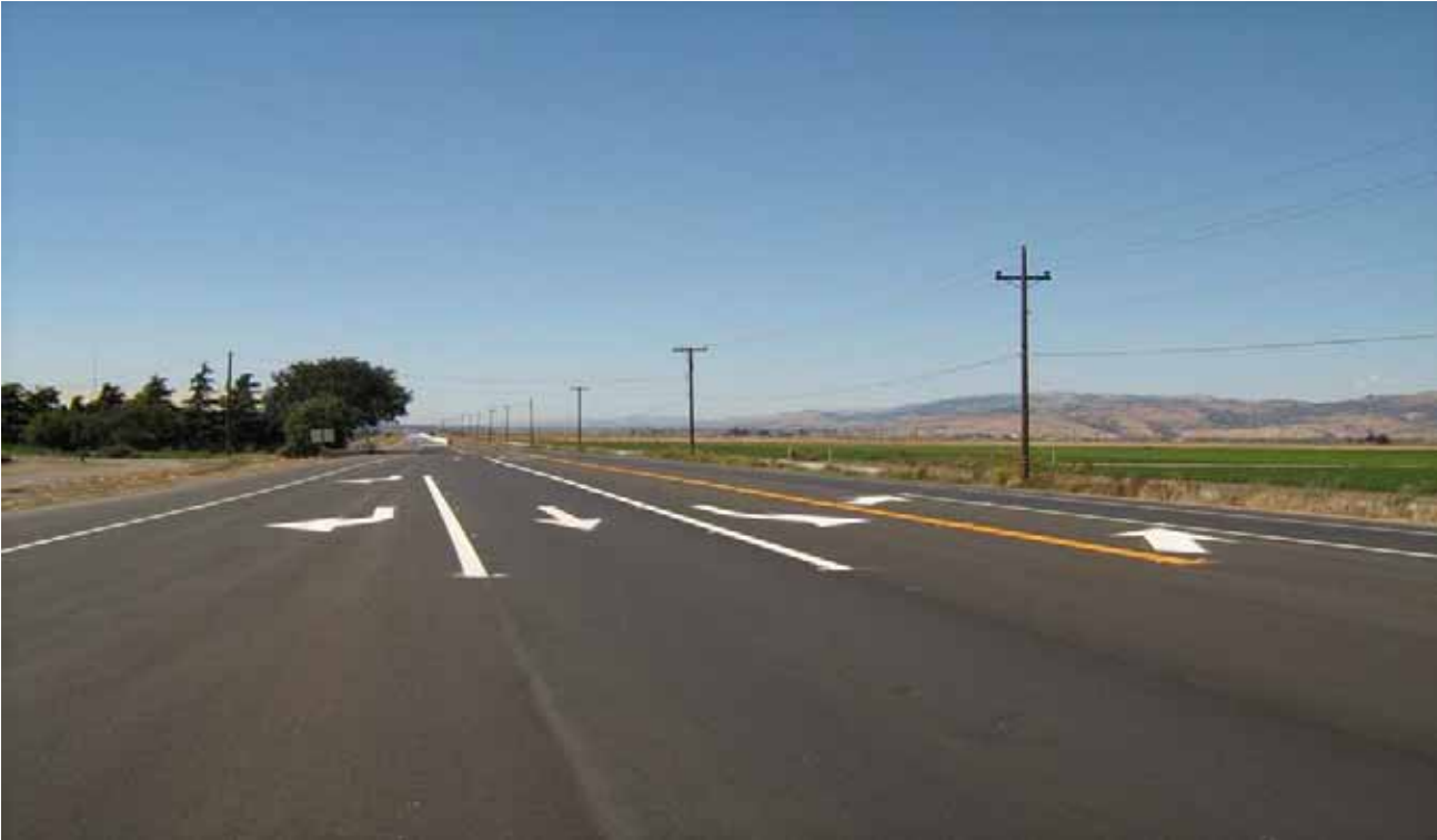
Intersection at Hudner Ln new Turn Lanes and Acceleration Lane
