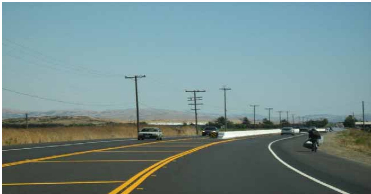
Final Stripe and Crash Cushion at Grant Line Rd.
